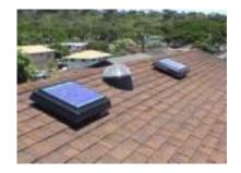
This small dentist's office has virtually no attic space to speak of. The whole building has a dropped ceiling with suspended a/c. In spite of being a brand new building, the Air conditioning could not keep up. Three fans for this 4500 square feet of roofing did the job.
